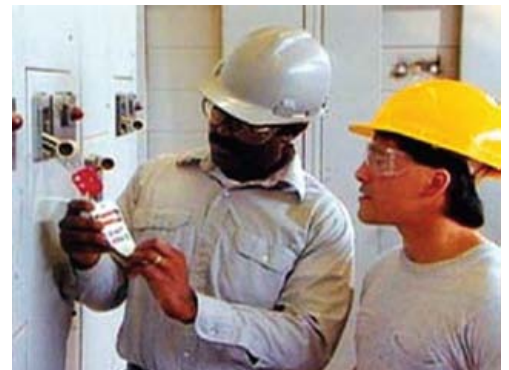
LOTO process used appropriately
